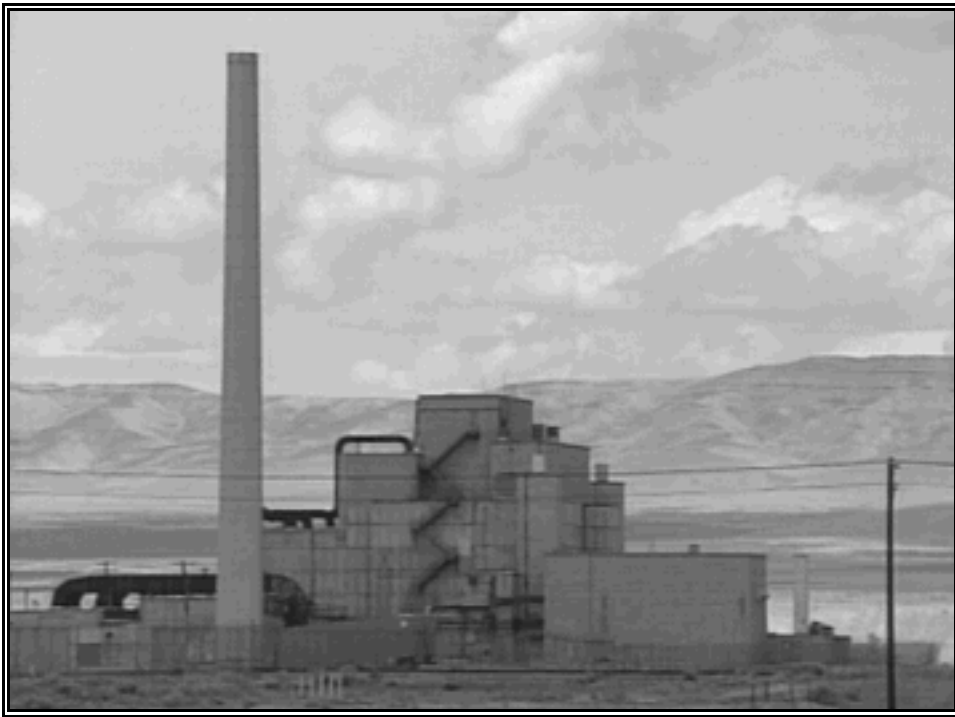
Fig. 12. D-Reactor, looking north, across the river to Wahluke Slope [DOE archive].
