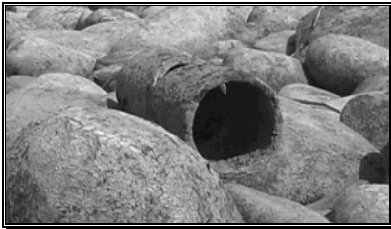
Fig. 8. Vent on top of D/DR-Reactor discharge pipe, upstream of D-Island.
