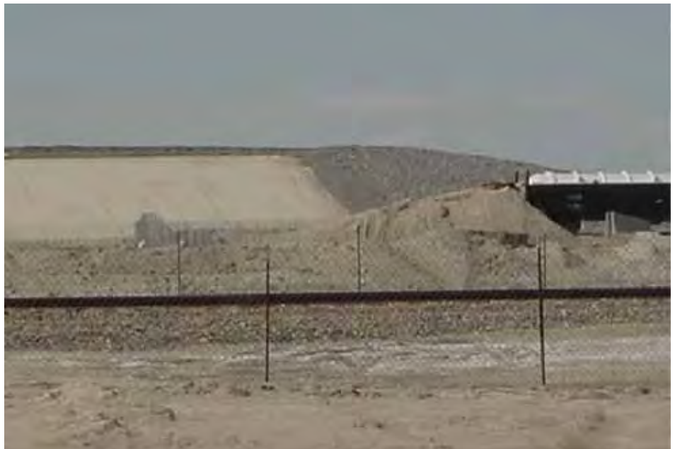
LARW Waste Embankment Cell
