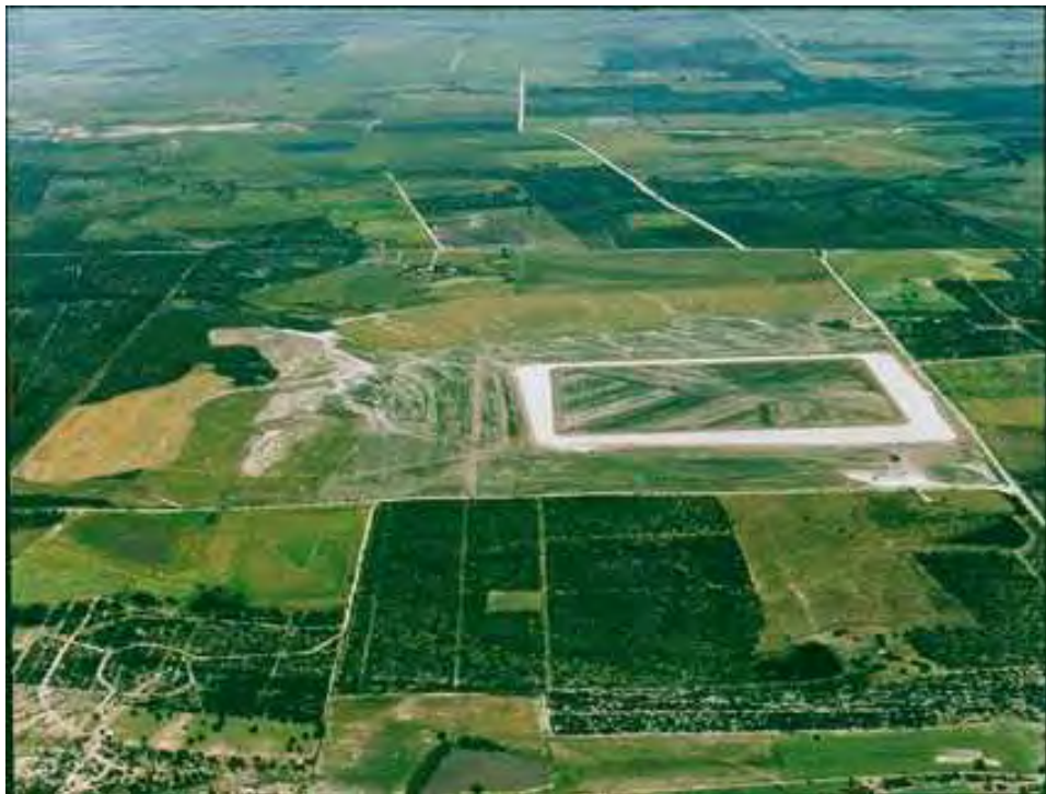
PHOTO 6 – Falls City, TX UMTRAP Site following surface remediation in place, 1994
